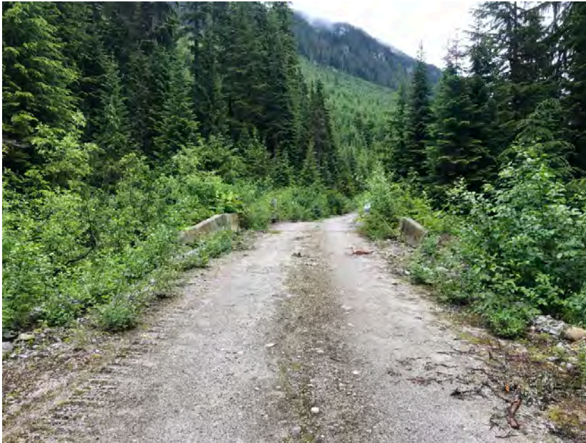
Approach from Right Bank when facing downstream
