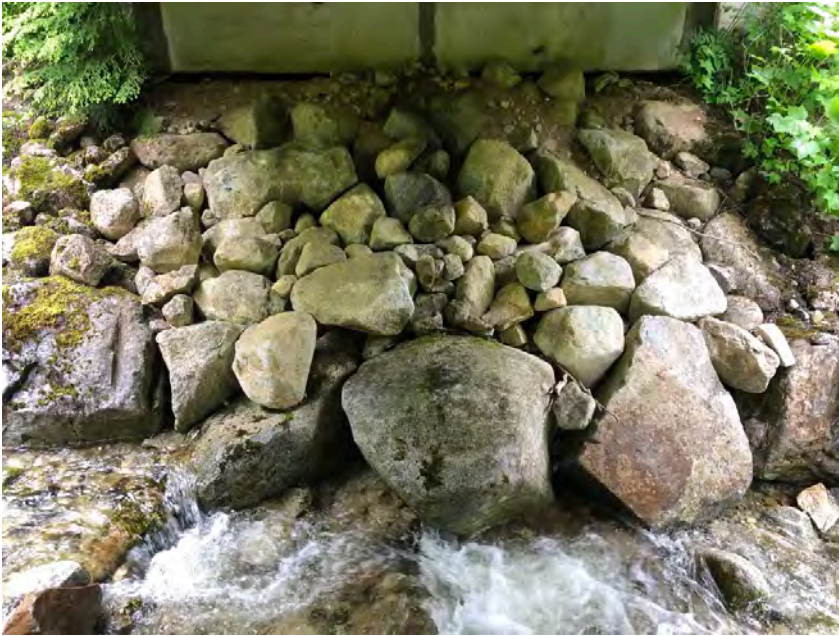
Left Bank Abutment when facing downstream
