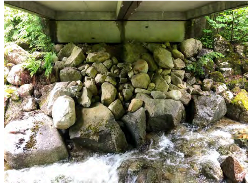
Right Bank Abutment when facing downstream
